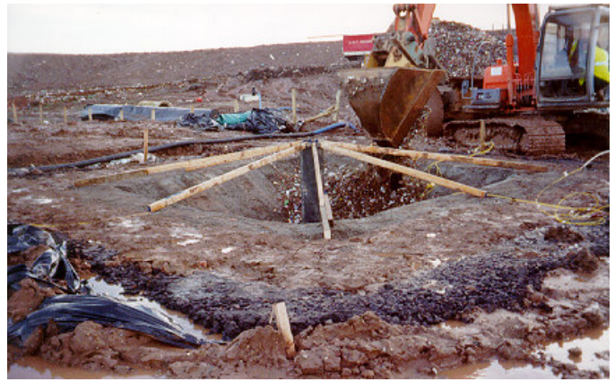
Figure 11 The completed experimental liner system, prior to filling and covering
